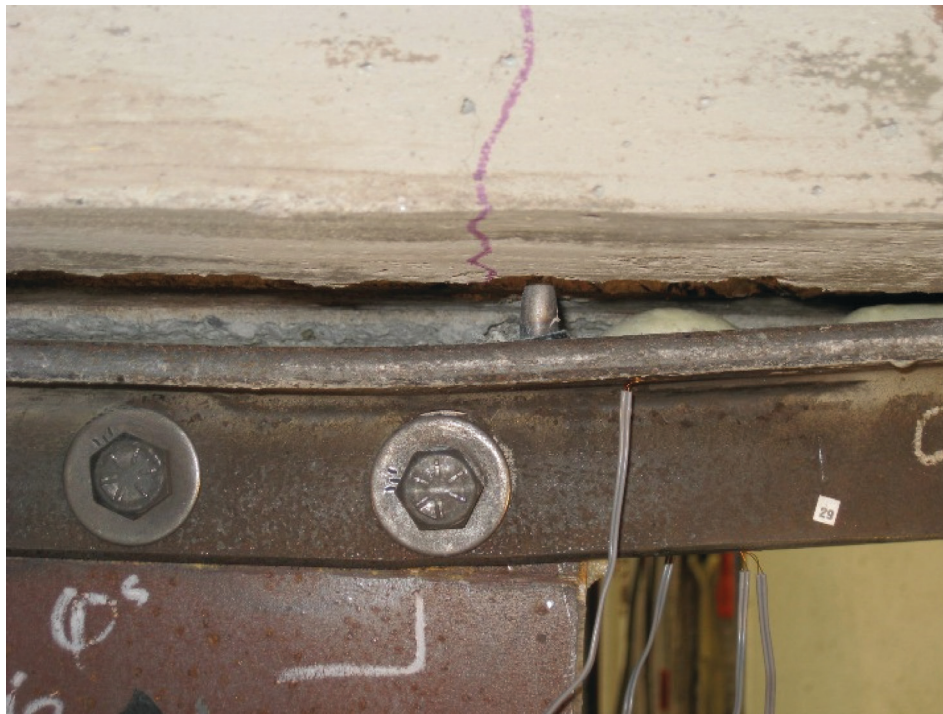
Fig. 20. Specimen F0B: rupture of stud connectors near the end of the top chord.
