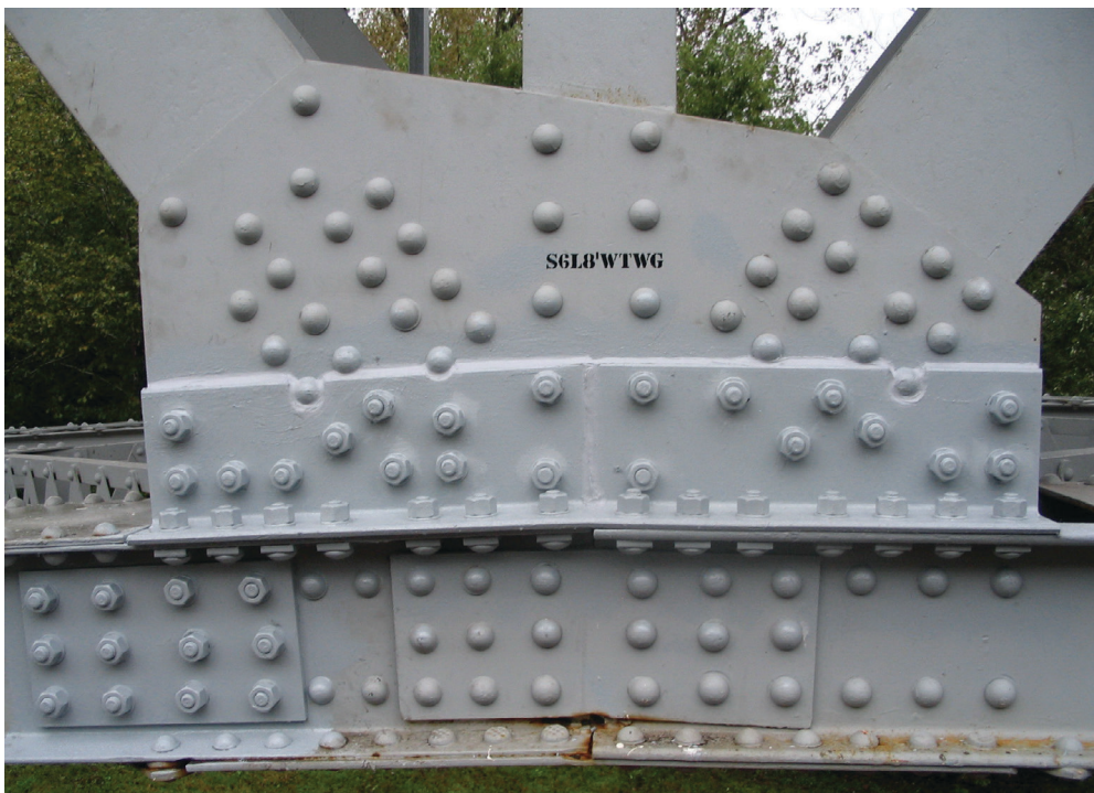
Fig. 11. Efficient repair addressing BCN deterioration.
