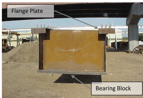
Fig. 4. Girder end to be embedded in concrete diaphragm.
