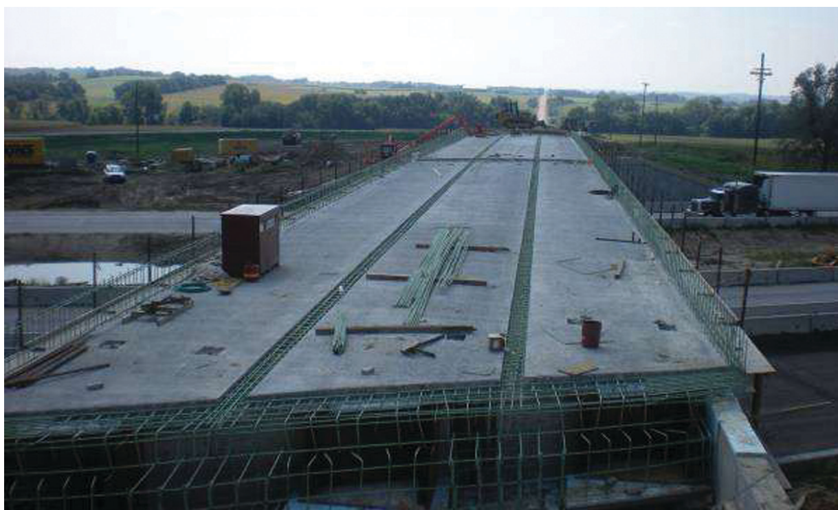
Fig. 25. Before casting the closure regions.
