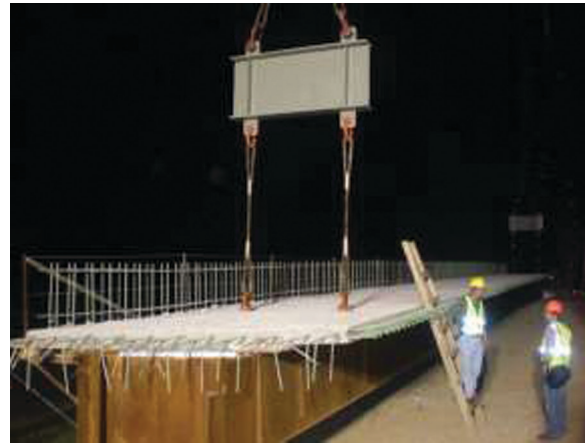
Fig. 21. Lifting of a single pre-topped girder for the 262nd Street Bridge.
