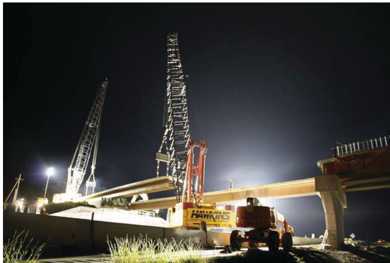
Fig. 22. Second girder in second span of the 262nd Street Bridge.
