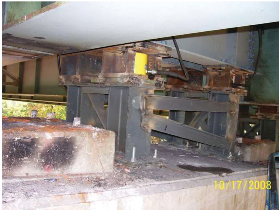
Fig. 8. Jacking and temporary support of bridge for bearing replacement.
