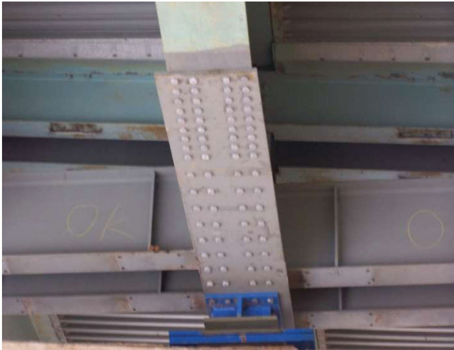
Fig. 6. Bottom-flange cover plate with skewed bolt lines.
