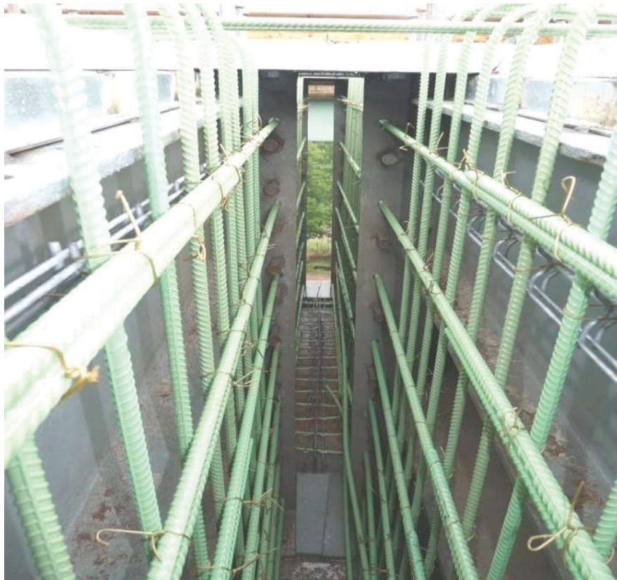
Fig. 7. Reinforcing and shear studs on stringer webs for full-depth concrete diaphragm.
