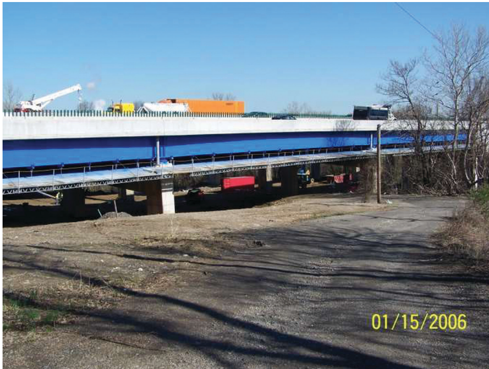
Fig. 11. Completed northbound three-span structure.
