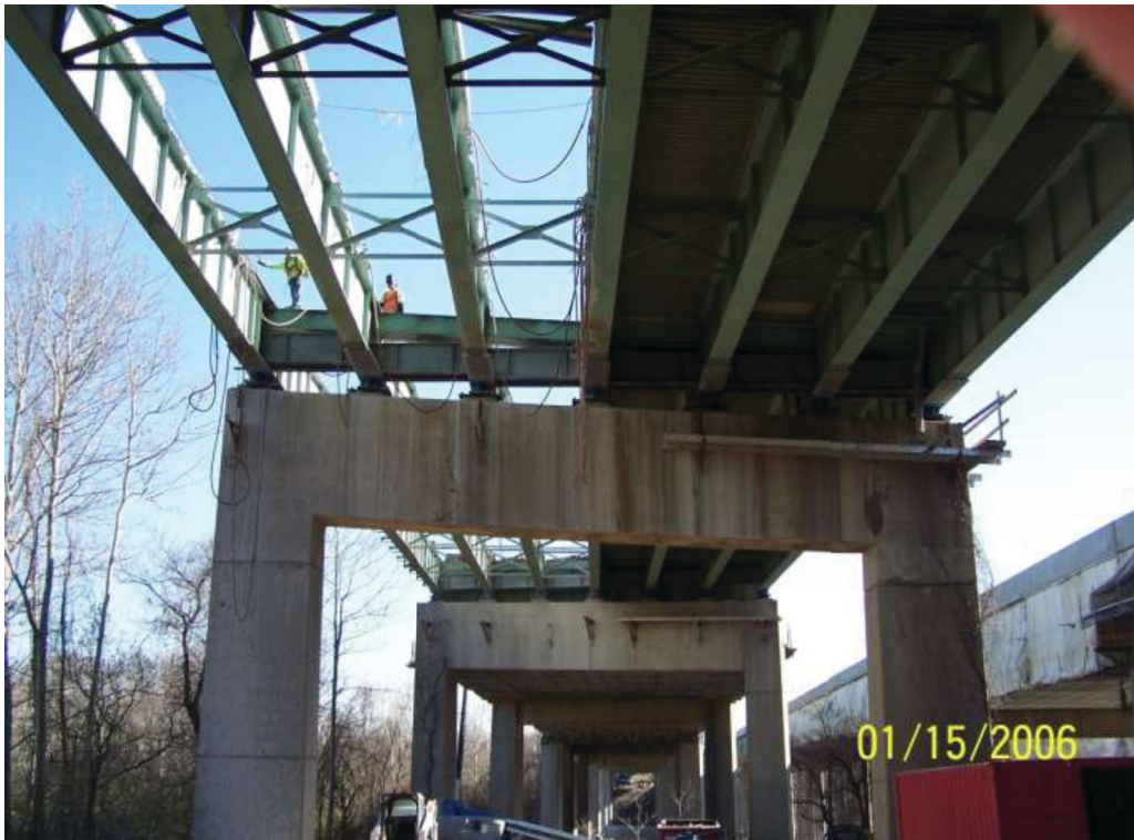
Fig. 2. Approach spans: seven-stringer cross-section during half-width redecking.
