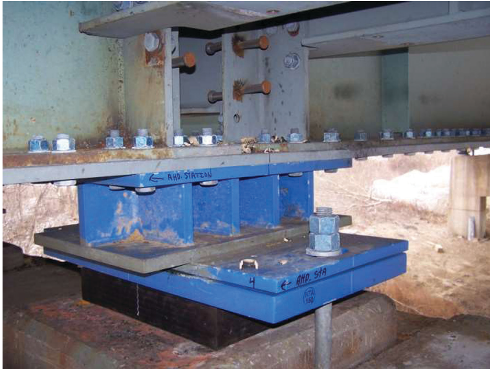
Fig. 9. Elastomeric bearings with steel bolsters.
