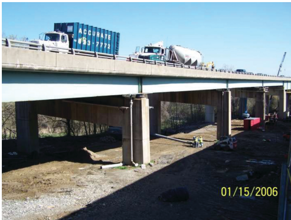
Fig. 3. Southbound approach spans: existing simple-span condition.
