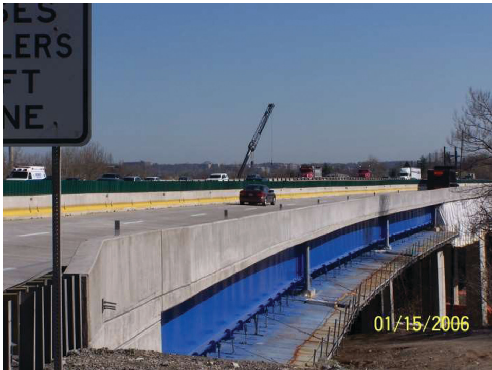
Fig. 12. Reduced number of deck joints.
