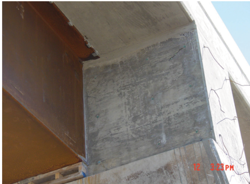
Fig. 12. An example of cracking in the concrete diaphragm if it is cast full depth.
