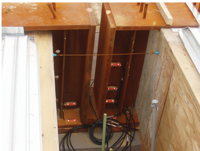
Fig. 11. Typical live load continuity detail used in field application; overall view on the left, close-up view on the right.
