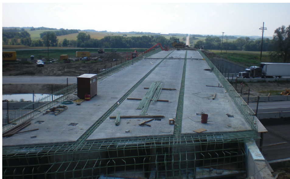
Fig. 18. Completing the placement of the pre-topped units for the bridge over I-80 at 262nd Street in Nebraska.
