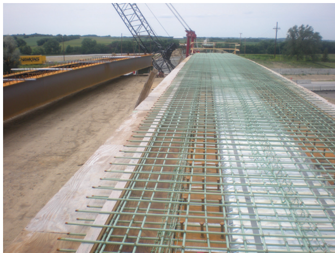
Fig. 20. Possible detail for longitudinal closure pour.
