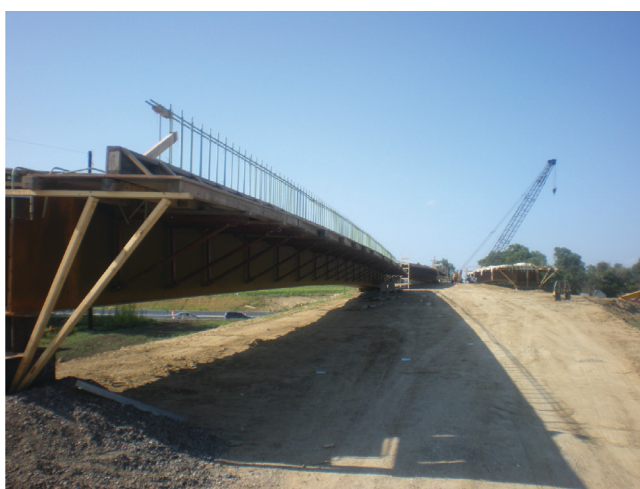
Fig. 16. Preparing the formwork for casting the deck on the unit.
