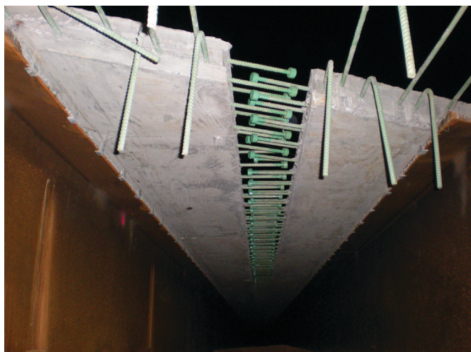
Fig. 20. Possible detail for longitudinal closure pour.
