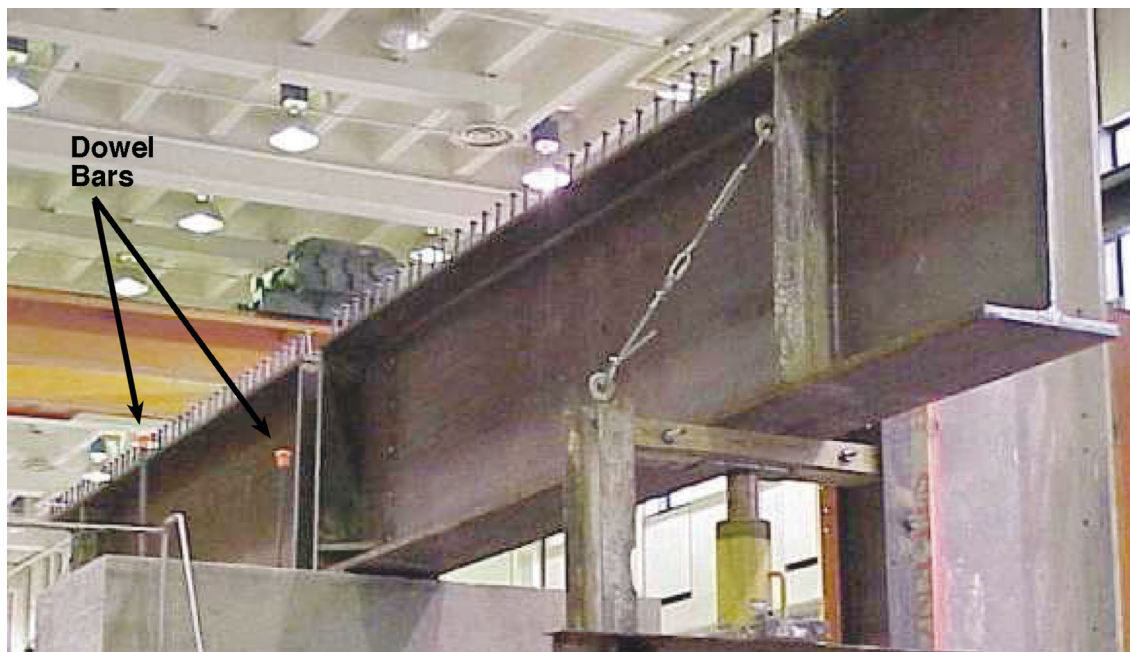
Fig. 5. Photo of the two girders during construction.
