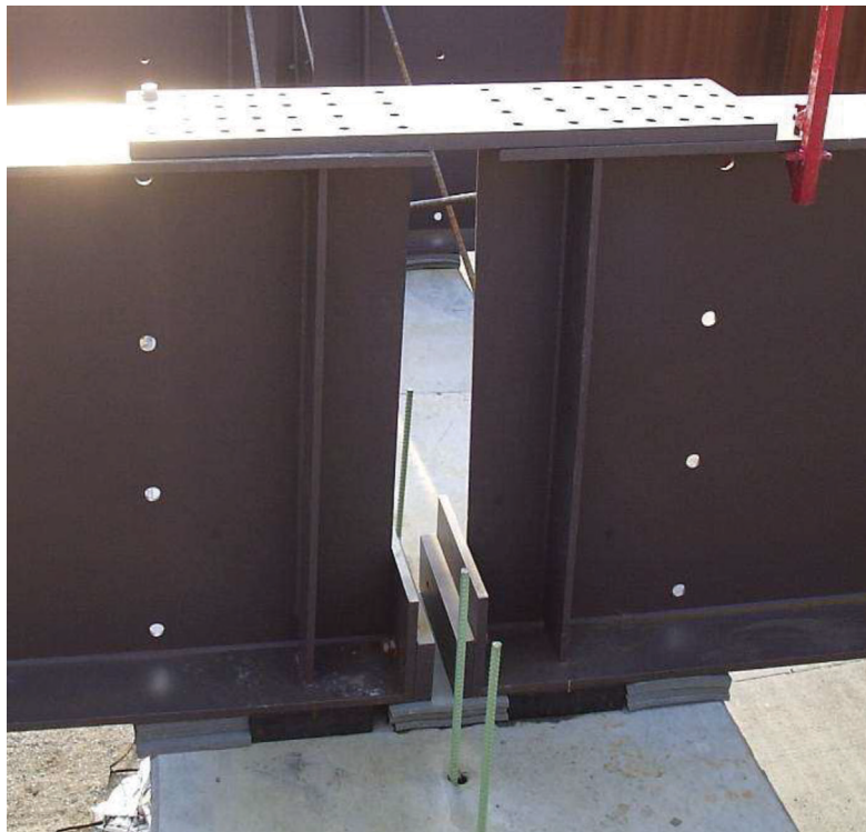
Fig. 6. Three Springs Drive continuity splice.
