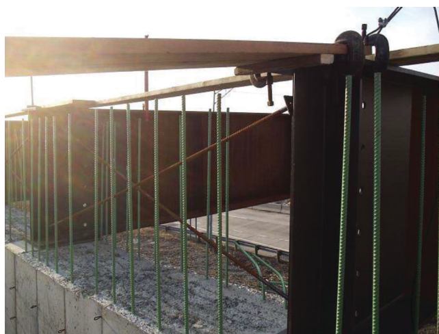
Fig. 8. Temporary cross frames at supports.
