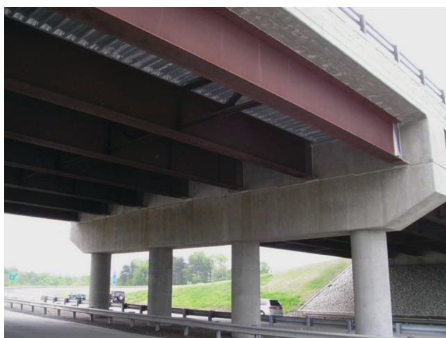
Fig. 7. Completed diaphragm.
