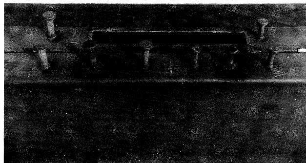
Fig. 5. Air supply hole in top of beam
