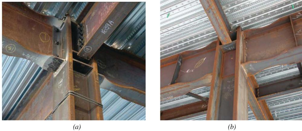
Fig. 1. RBS moment connection: (a) with continuity plates; (b) without continuity plates.
