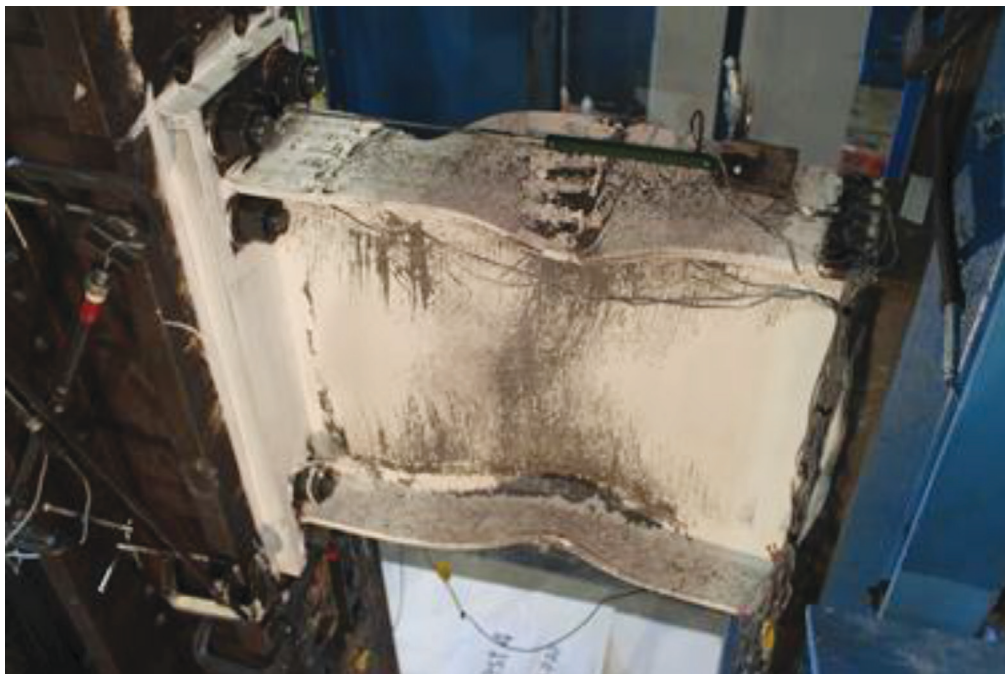
Fig. 5. Deformed protected zone with intermittent powder-actuated fasteners in the flange (photograph courtesy of Professor Matthew Eatherton).
