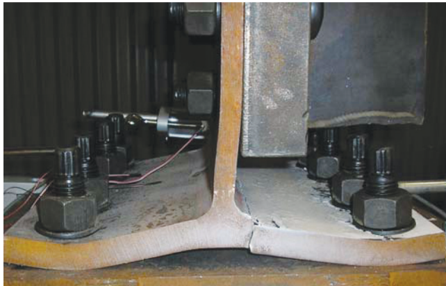
Fig. 13. Example phase 2 flange fracture location.
