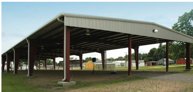
Fig. 1. Example of small open-building application.
